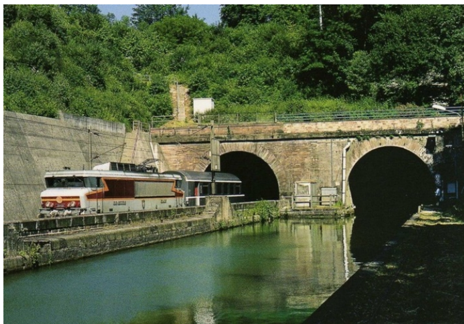
Photo : Arzwiller tunnel
